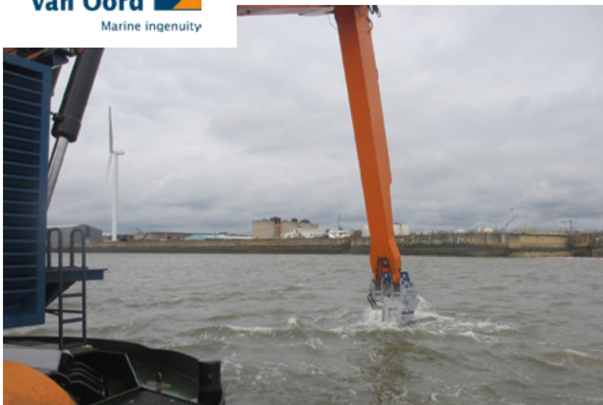
Model: XR80 – Project: Dover harbor UK, July 2013
